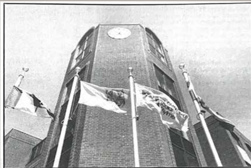
The three-year-old Place des Pionniers building is home to Aylmer city hall, the Aylmer School Commission, Travail Québec and regional government branch offices, provincial MNA Robert Middlemiss's riding office and assorted businesses
