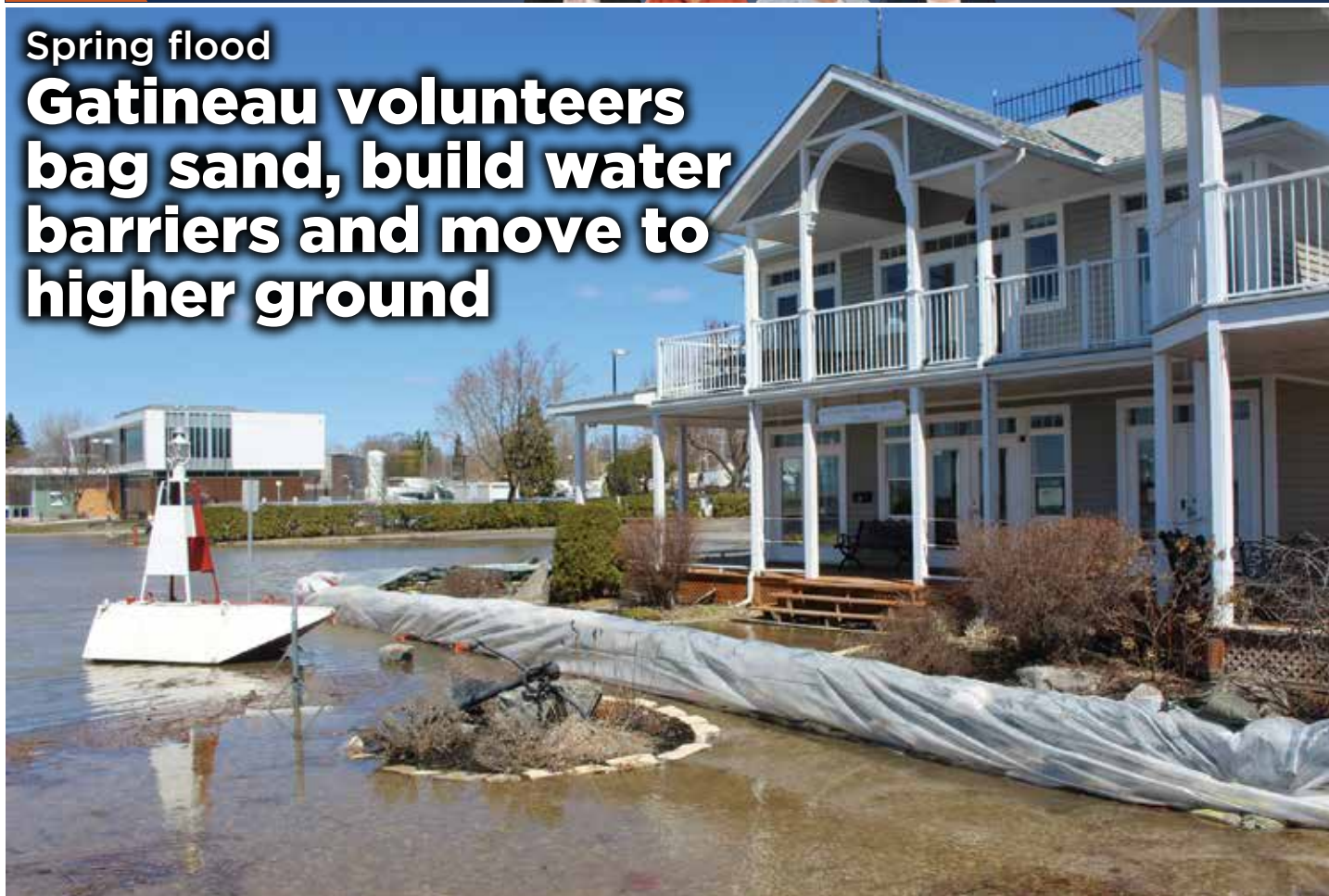
The Pavilion Robert-Middlemiss and the Water Treatment Facility were also protected in case water levels rise further. (SD)
